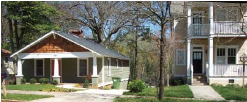
A zero-step entrance (at left) makes homes more easily accessible to people with mobility impairments than the conventional multiple step entrance (at right).
